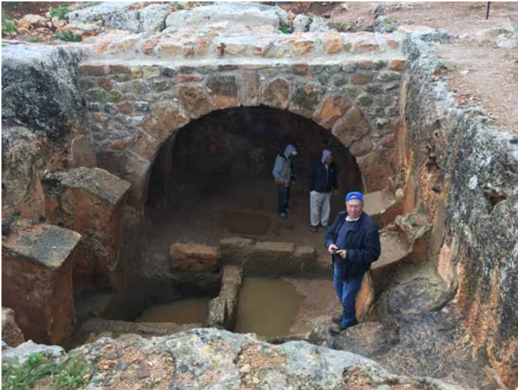
Fig. 10.16. Reconstruction of two arches and roof slabs on the eastern side of the Large Arched Reservoir.
